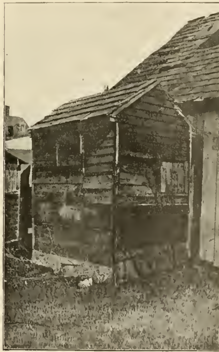
ORIGINAL TICKET OFFICE OF THE NEW CASTLE & FRENCHTOWN RAILROAD, BUILT 1832.
